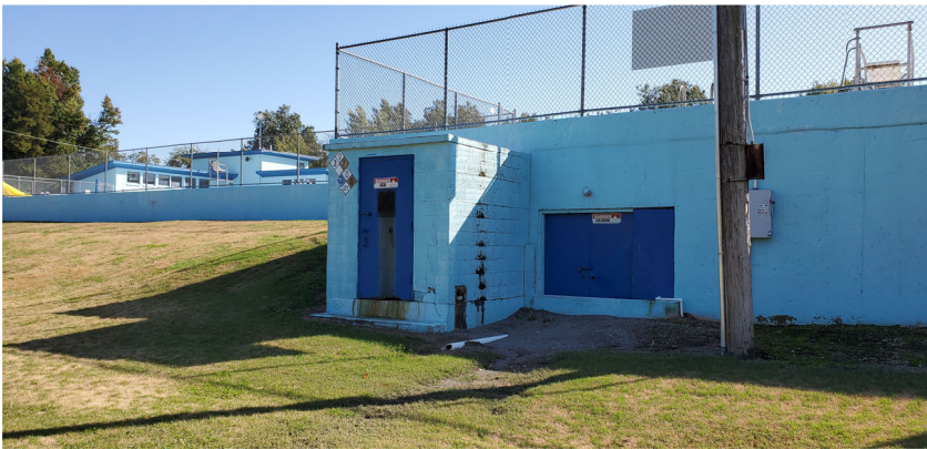
Chemical storage building.
