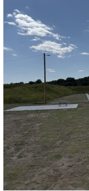
Final rifle-range concrete pad
