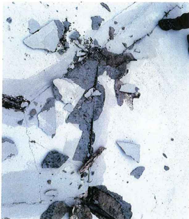
Figure 3 CLOSE UP OF WEATHERED JOINT
