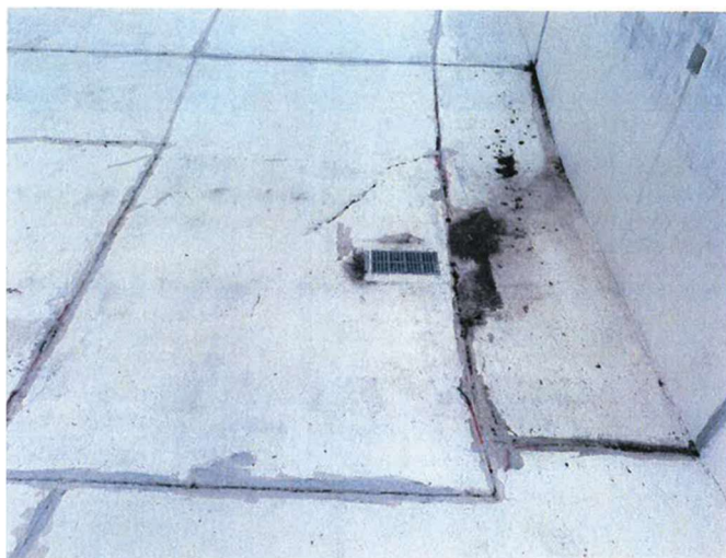
Figure 3 CLOSE UP OF WEATHERED JOINT
